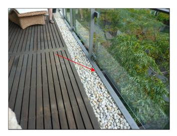
The balcony is partially covered with a timber deck which is bordered by white/light coloured pebbles of various sizes. The pebbles are laid loose on three sides of the balcony directly onto the slab to a depth of approx 75mm. In general, the pebble finish is level with or slightly above the rail edge (arrowed). There is a gap of approx 50mm between the upper edge of the rail and the glass panels.
