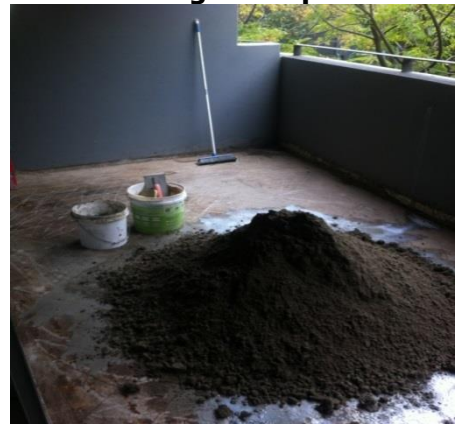
Screed being laid Apt. 317
