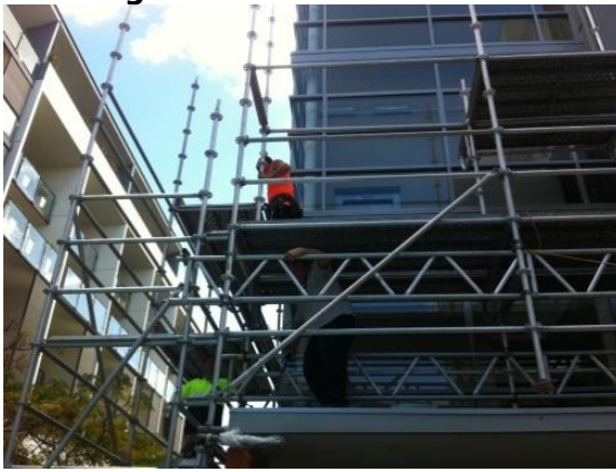
Building 2 scaffold installation
